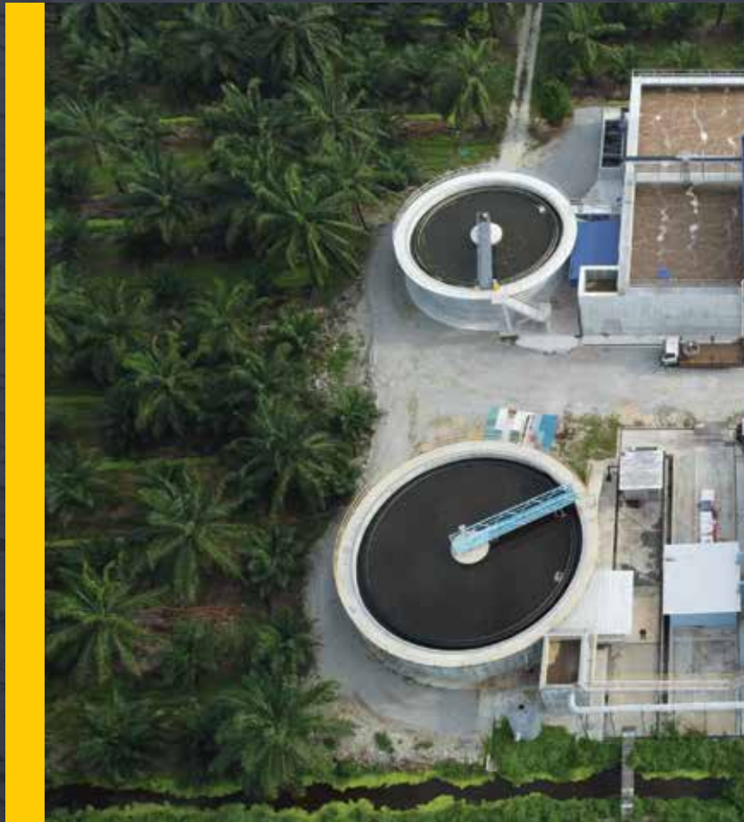
Biological Nutrient Removal (BNR) Technology at Seafood Processing (5,000 m 3 /d)
