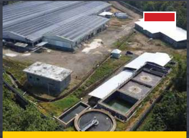
3,000 m 3 /d Chicken Processing WWTP
