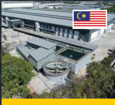
1,000 m 3 /d F&B WWTP
