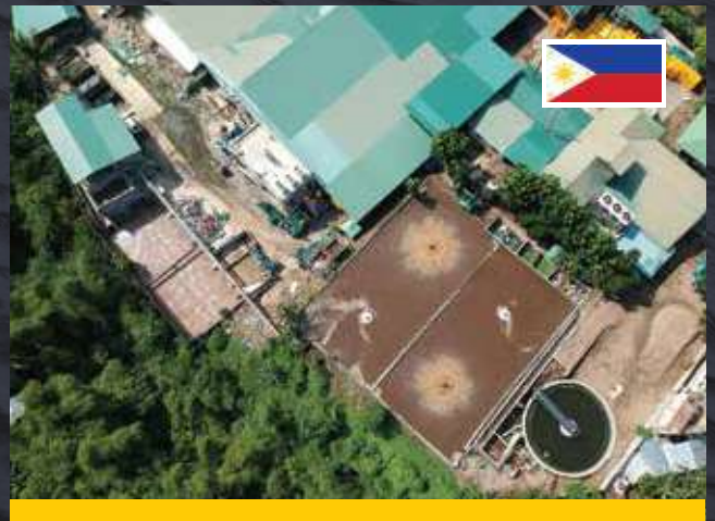
2,000 m 3 /d Chicken Processing WWTP
